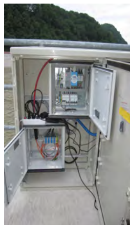
Heating modules on the left and reading units and modem on the right
