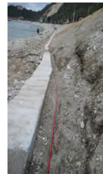
Sava river near Krško on the left and hybrid DTS cable during installation
