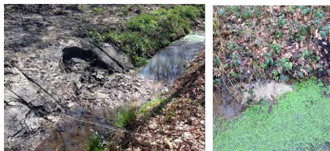
Slope instability and sand boils in a ditch along the canal
